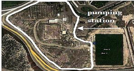
Fig.1. Location of Water Pump Station.
