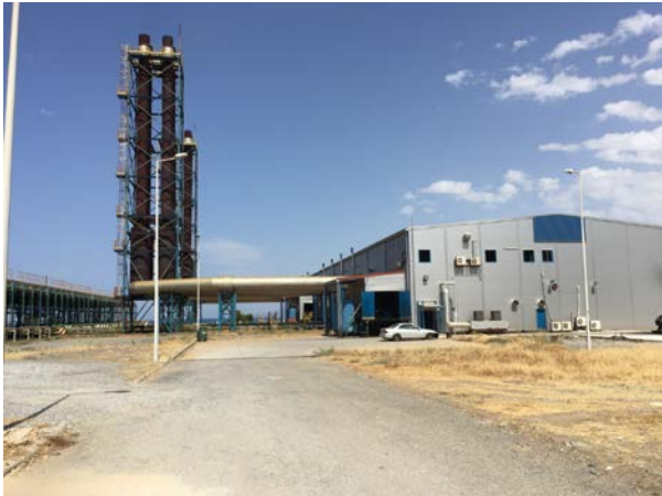
Figure 1. Diesel Generator Section of Tekneçik Thermal Power Plant.
