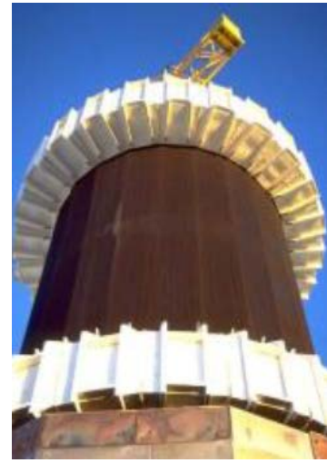
Fig. 1. Solar Two receiver [10]
